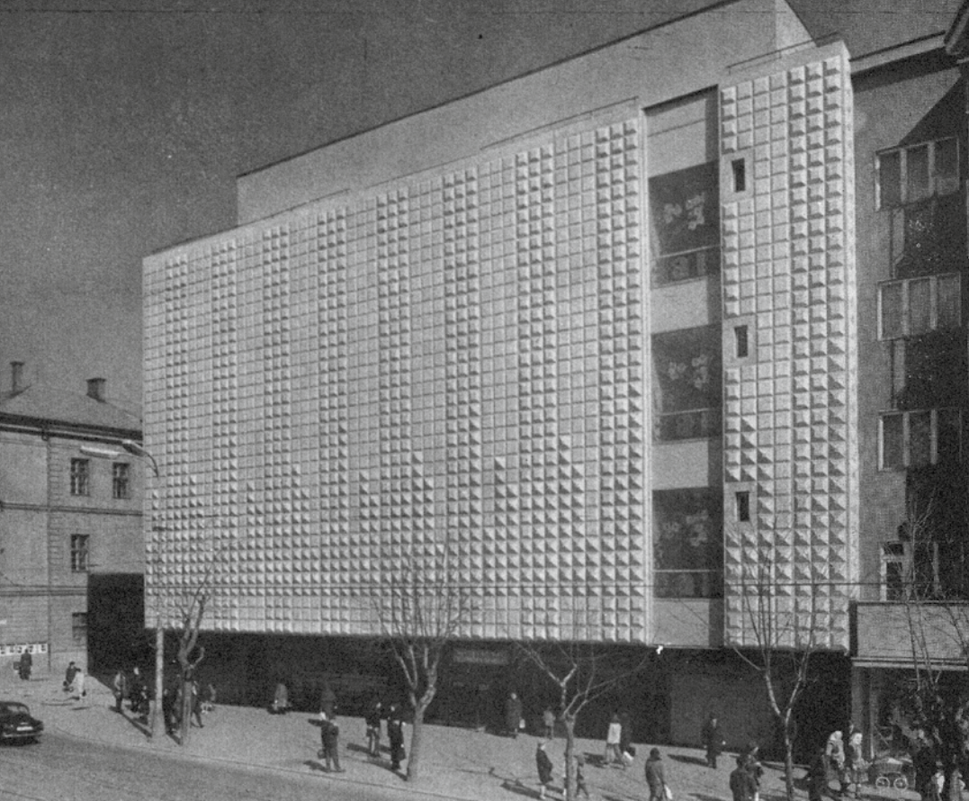
THE WEST FAÇADE, VIEW FROM HLAVNÁ ULICA.
