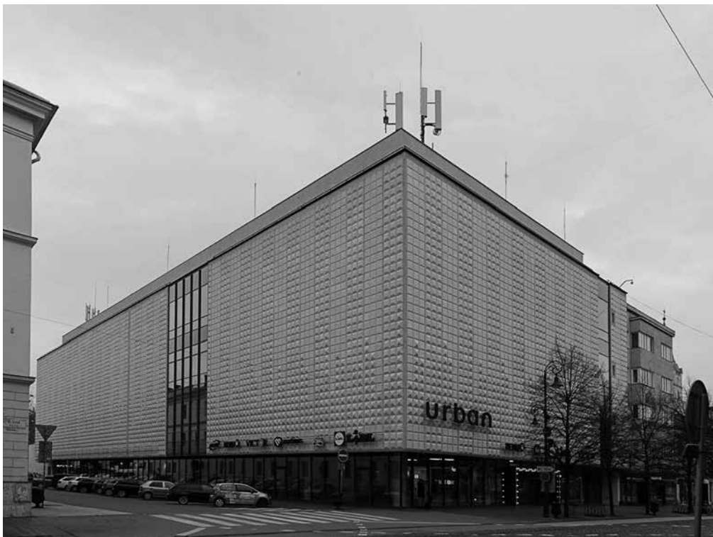
CURRENT STATE OF THE FAÇADE, AUTHORS OF THE RECONSTRUCTION: ABMV WORLD, PRAHUE; M-PROJECT, POPRAD, 2020 – 2021
